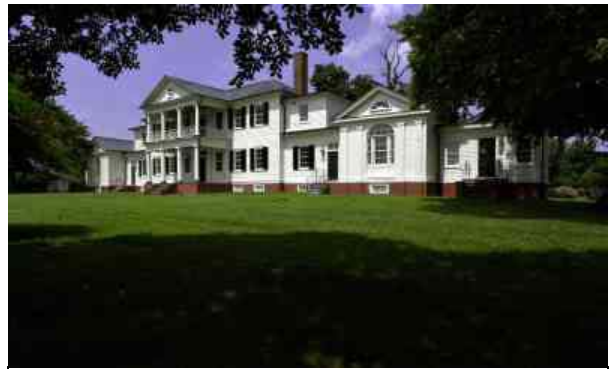
The riverfront entrance of Belle Grove, built around 1790, shows the restored home that occupies the property once owned by the family of James Madison, the nation's fourth president, who was born in a house nearby in 1751.
